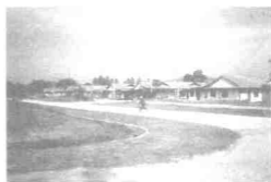
A low cost housing in Kupang
